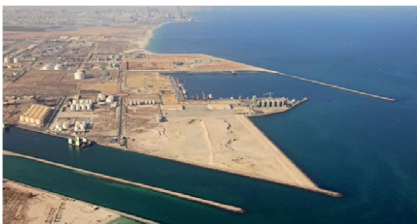
The port of Hamriyah in Sharjah. (Sharjah Ports)
