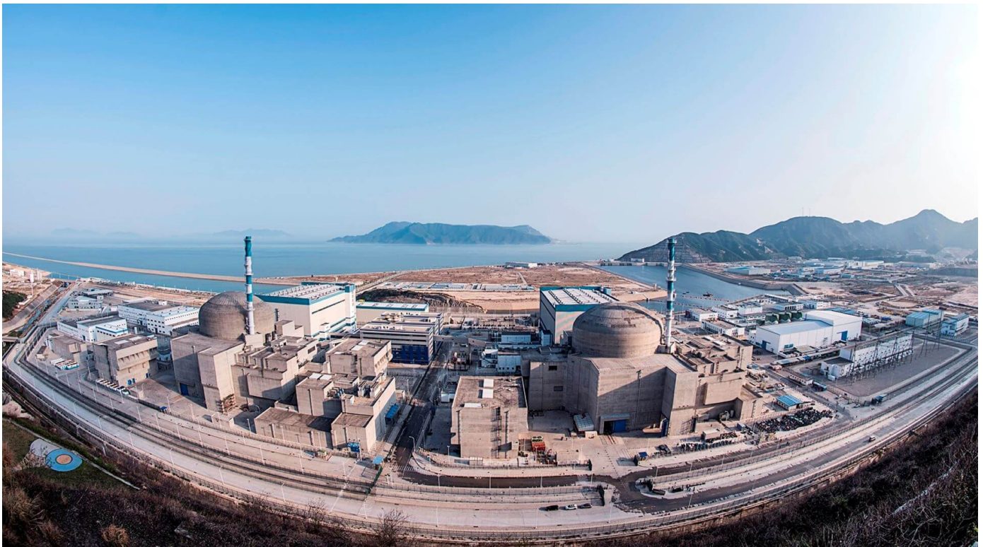
▲ Taishan nuclear power plant, Guangdong, China
